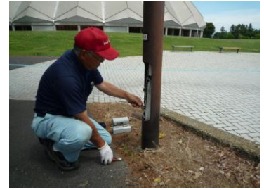
LED 用電源機器取付
